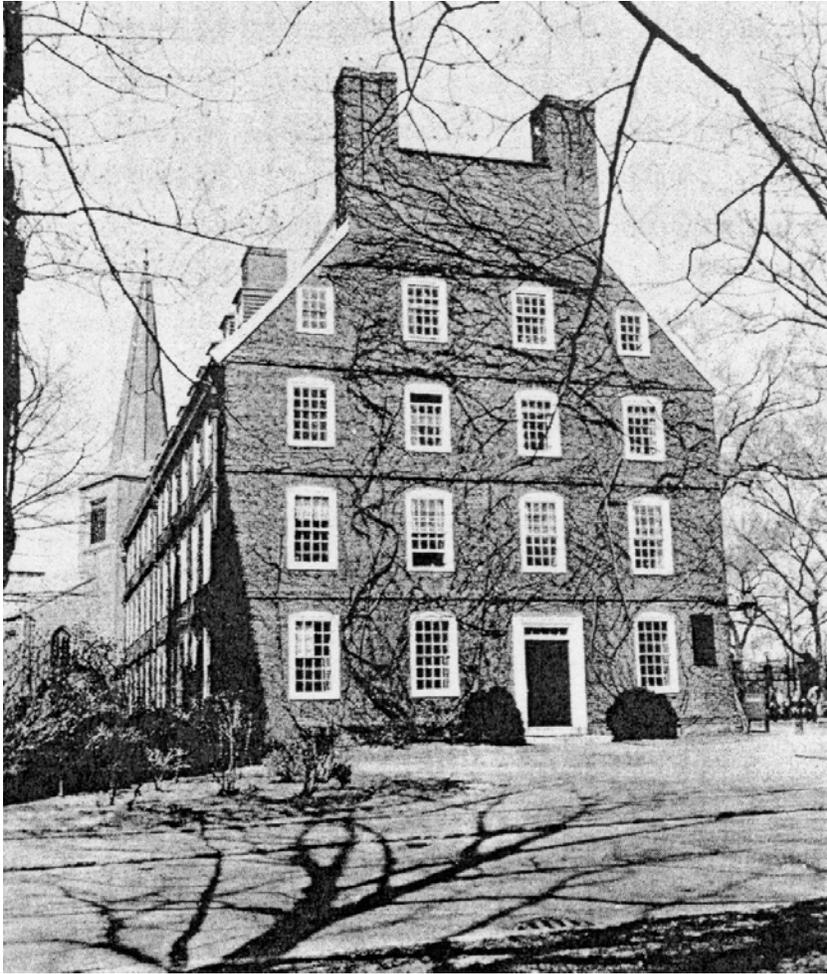
Figure 3. Historic Massachusetts Hall at Harvard University was built in 1720 with straight lime/sand mortar, and has never needed re-pointing [photo from Speweik].
